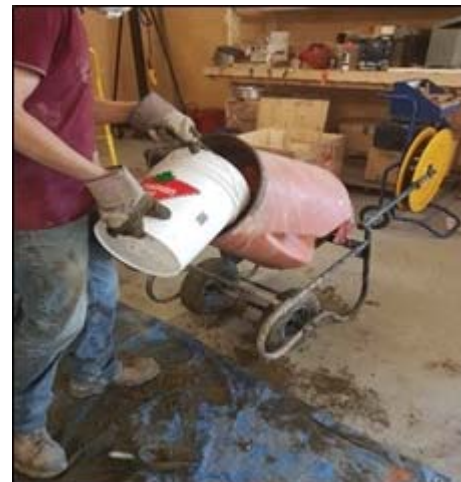
Figure 3. Concrete batch mixing using a portable mixer
